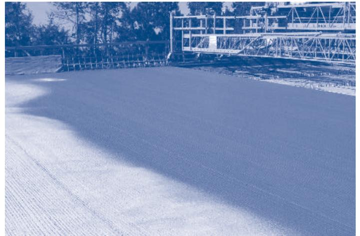
*150 pcy ICC placement (note the lack of curing compound on the right)*
